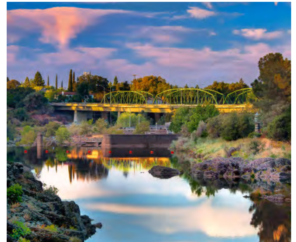
The tranquil nature of the pool upstream of the Fish Barrier Dam reflects the Table Mountain Bridge and downtown Oroville.
