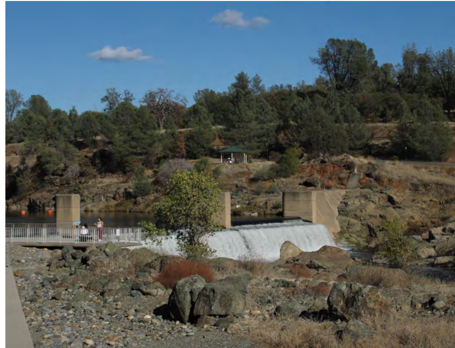
View of the Fish Barrier Dam from Downstream
