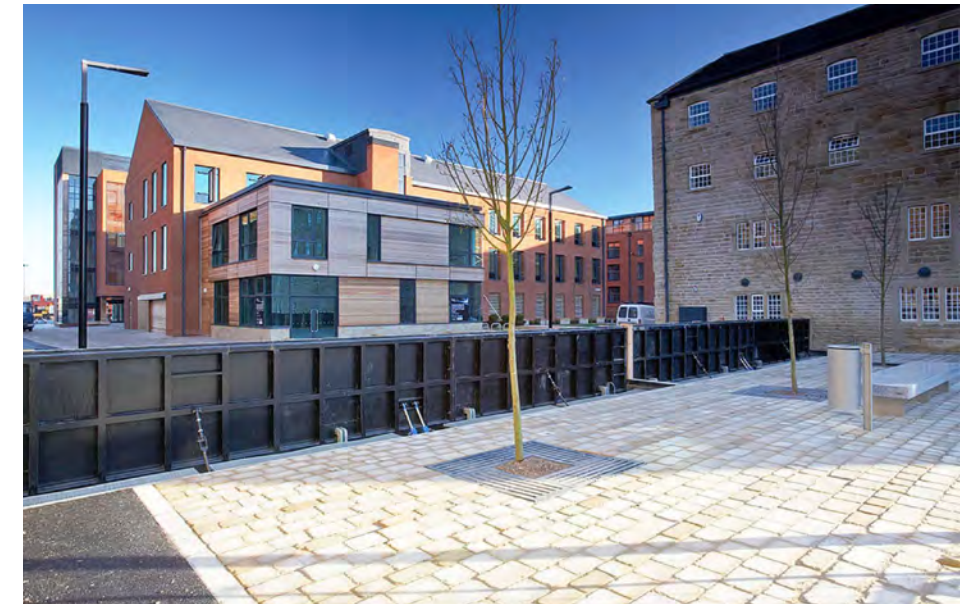
Flood protection and development can be fully integrated into functional and inspiring landscapes suitable for living or working. This includes operable barriers that stay hidden except for during floods.
