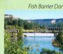
Fish Barrier Dam
