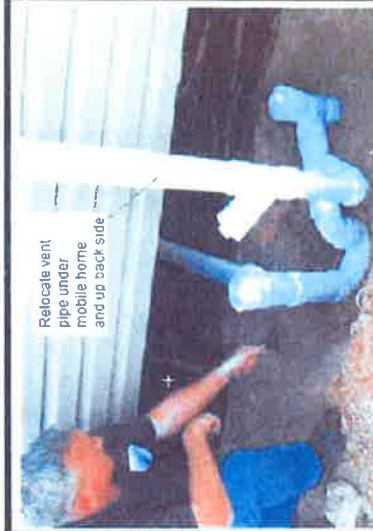
SEWER LINE VENT PIPE AND CLEAN OUT DETAIL
