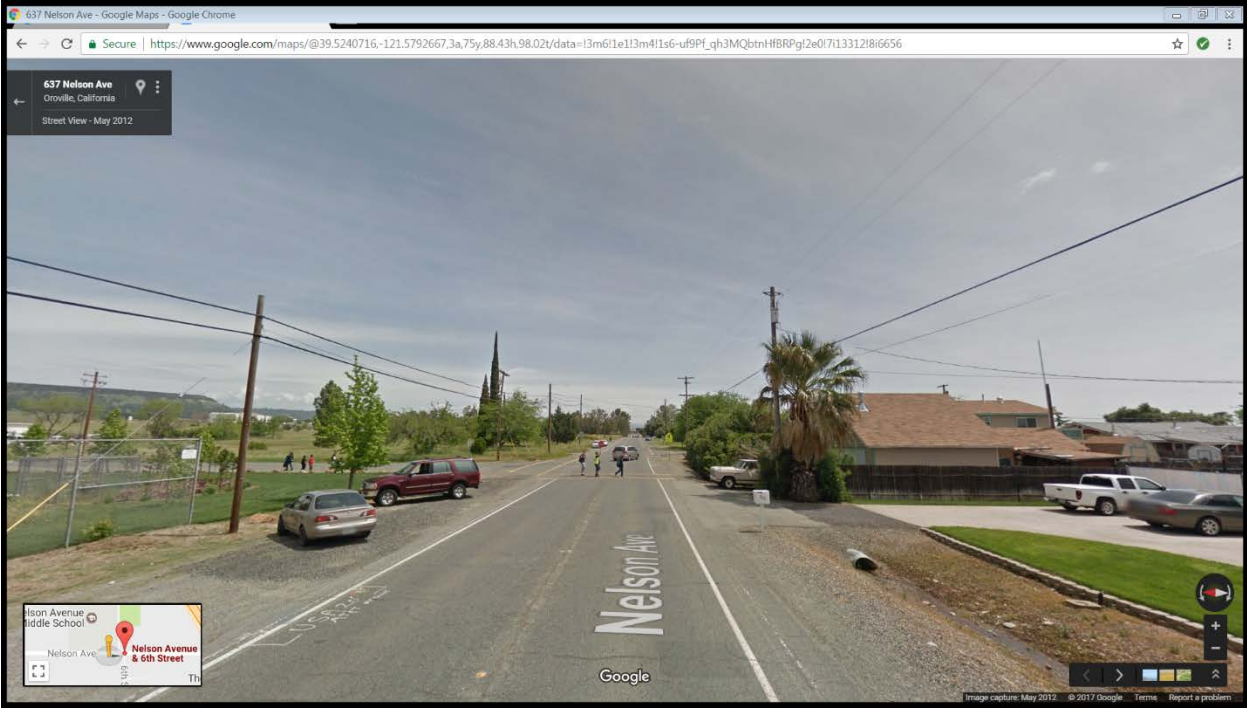
Above: Eastbound Nelson Ave approach to 6 th .
