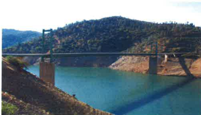
162 Bridge across Lake Oroville
