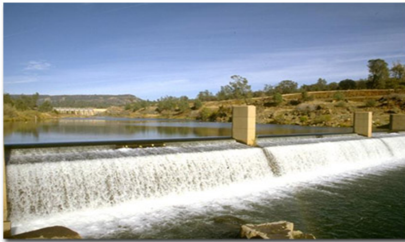
Diversion Dam near the Feather River Fish Hatchery
