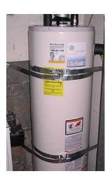
Prevent gas leaks and water damage during an earthquake by properly securing your water heater as outlined in this bulletin.
